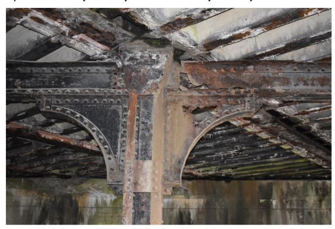
Showing 100% section loss, severe corrosion on the Freeport Bridge that could cause its collapse.
