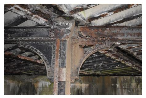
Severe corrosion on the Freeport Bridge could cause its collapse.
