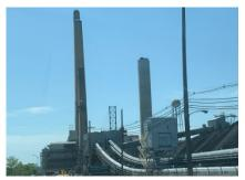
7. First Energy/W.H. Sammis Power Plant – A coal-fired power plant that includes 7 coal-fired units and five oil-fired units. The ponds are permitted to discharge into the Ohio River. The site contains 2 ponds to store bottom ash and wastewater produced by plant operations. The ponds are above the FEMA 100-yr flood elevation, and according to a report prepared by Geosyntec Consultants, the river has reached the toe of the embankments twice in the last 74 years.
