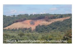
1. Revolution Pipeline explosion site – The location where Energy Transfer Partner's (ETP) natural gas pipeline exploded on 9/10/18. A landslide caused the explosion, which destroyed one home and damaged other nearby property. ETP has since failed to stabilize the land. Another pipeline currently under construction will cross the Revolution's path less than 500 feet from the explosion to bring natural gas to the Shell Ethane Cracker. The Revolution pipeline crosses the Ohio River.
