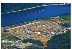
**11. Blue Racer Midstream Fractionation plant** – A plant that separates dry natural gas from natural gas liquids (NGLs), such as ethane, propane, and butane. The facility has recently applied to the WV DEP for a permit to modify the plant, involving increases in emissions.
